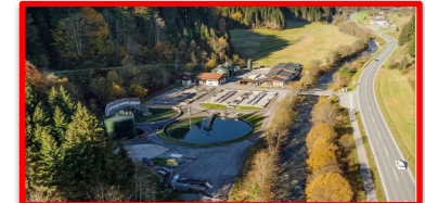
Waste Water Treatment
