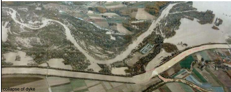
collapse of dyke
