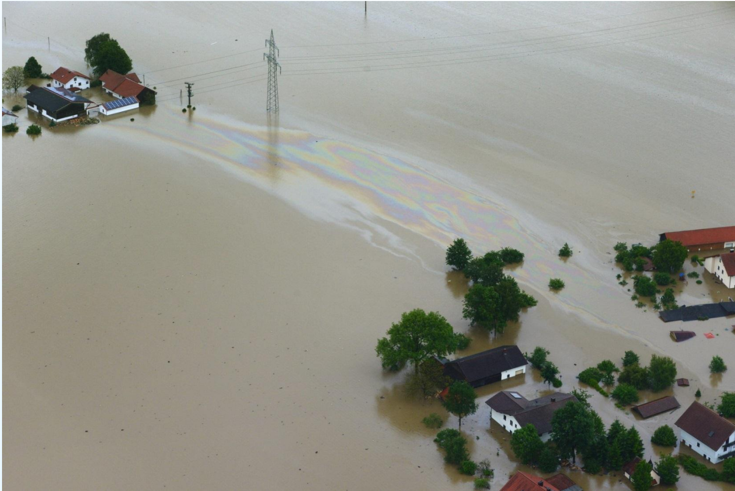
Flood 2013: oil leads to a total damage of houses
