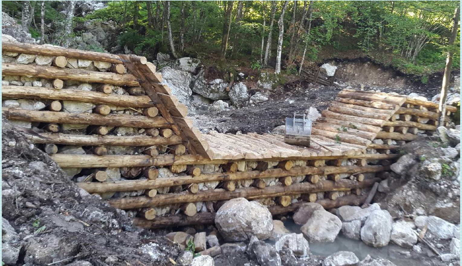
Torrent Suhi potok, realised by Hidrotehnik 2015 Photos: HIDROTEHNIK
