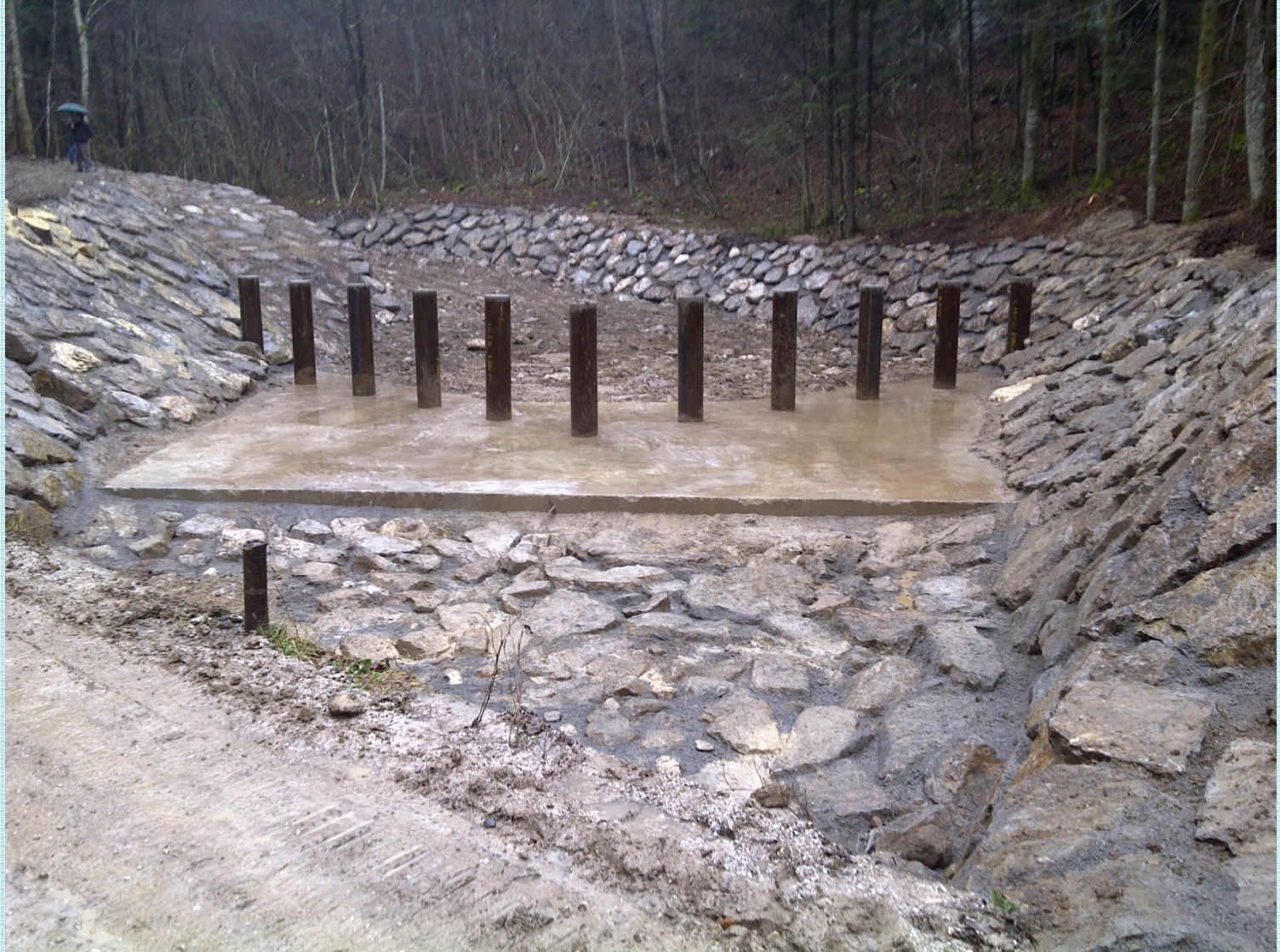
Torrent NIKOVA (2014); (measures for driftwoods); realised by Hidrotehnik 2015
