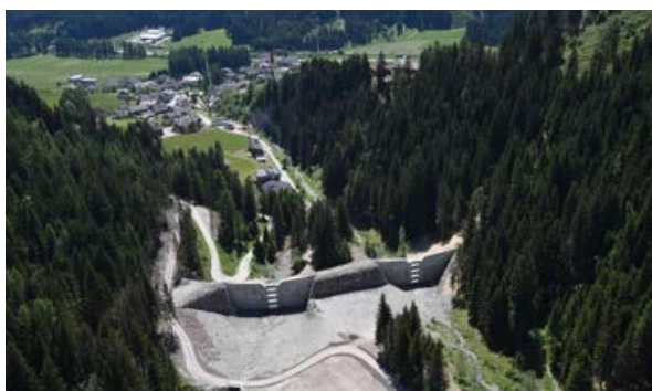
Figure 14 : Barrages de correction – Winnebach, Haut-Adige/Sud-Tyrol (© Province autonome de Bolzano/Bozen, Agence de la Protection civile)
