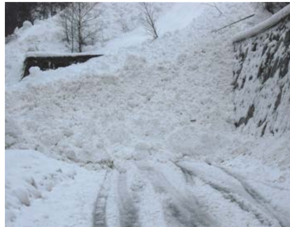
Figure 47: Example of deposition area that blocks the tunnel entrance (©Autonomous Region of Aosta Valley)
