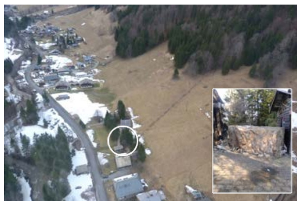
Figure 33: Rockfall in Morzine, Upper Savoy, 2013 (©National Forests Office, Land Restoration in Mountains)
