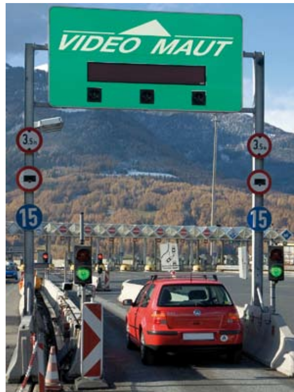
In Austria toll charges for motorcars are controlled by video (Source: ASFINAG).
