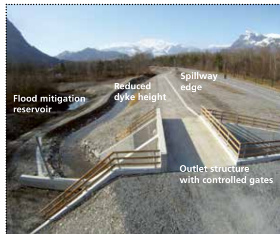
Figure 7 – Säga retention basin with controlled outlet structure and provision for the case of excess load for the controlled flooding of the dyke. (Amt für Wald, Natur und Landschaft)
