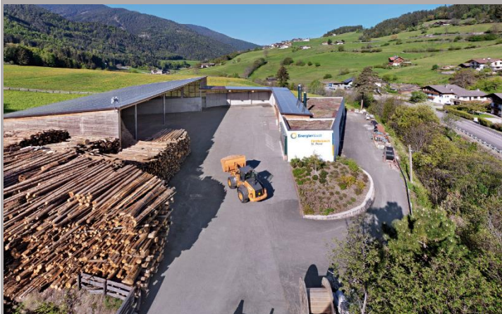
The biomass district heating plant. Source: Energy cooperative Villnöss
