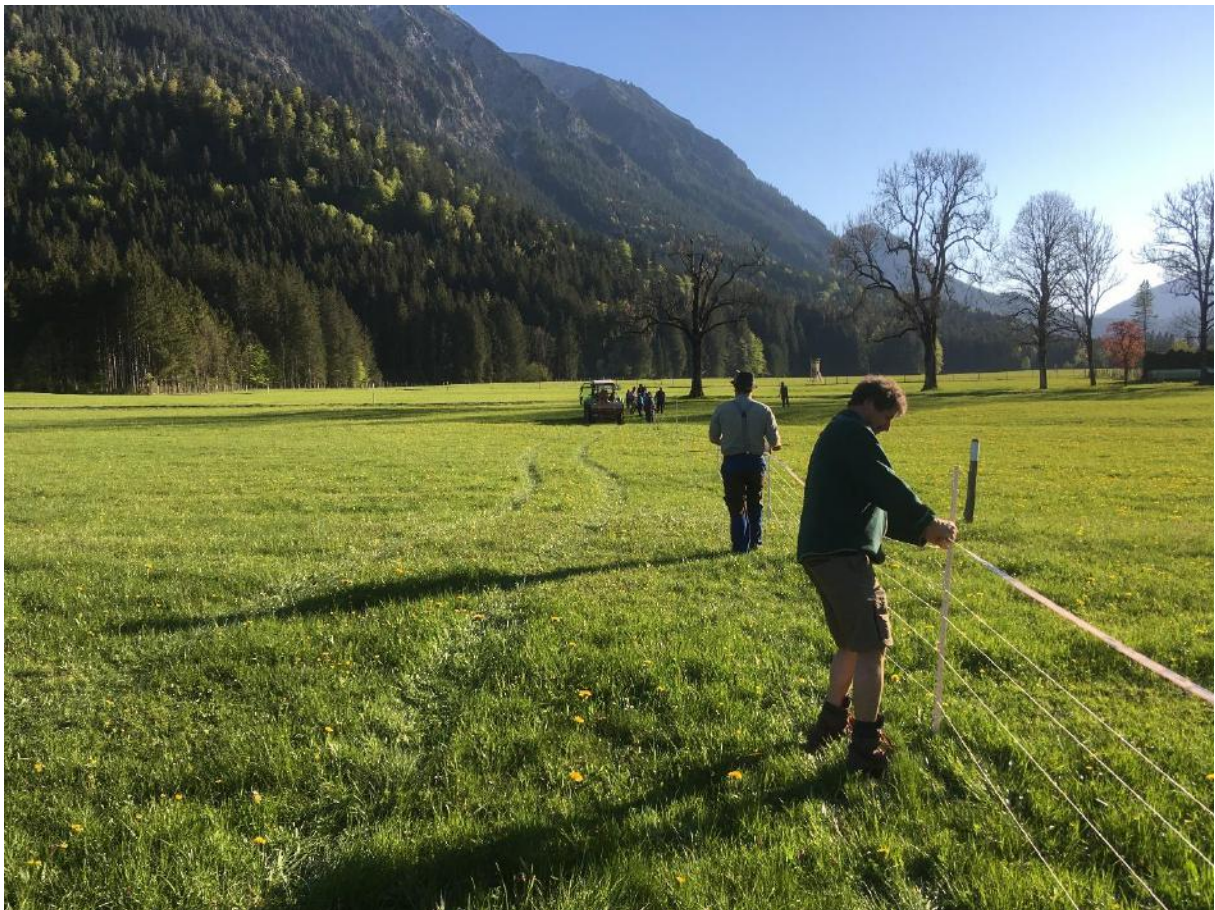
5-wire electric fence (120 cm height), damage prevention due to bear presence.
