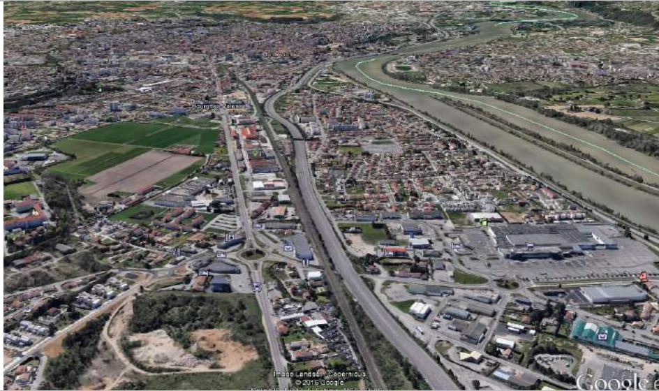
Illustration 43: A7 Tain l'Hermitage – Valence Sud. Aerial view (GoogleEarth) of the area close to Valence.
