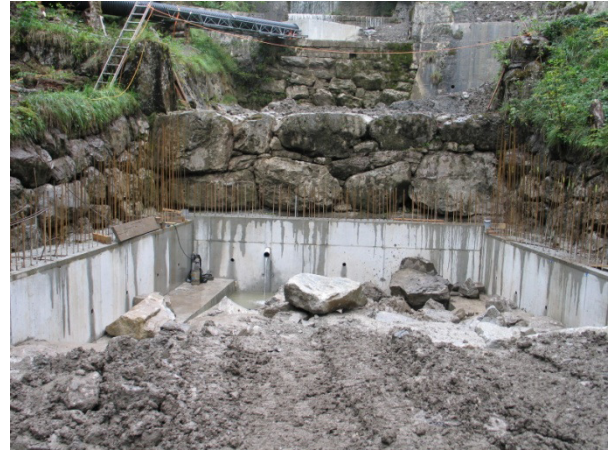
Pre-concreting and training structures
