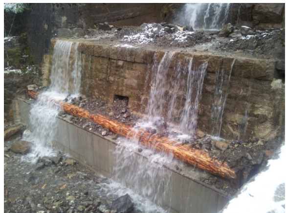
Finished pre-concreting and coverage with log Source: canton of NW
