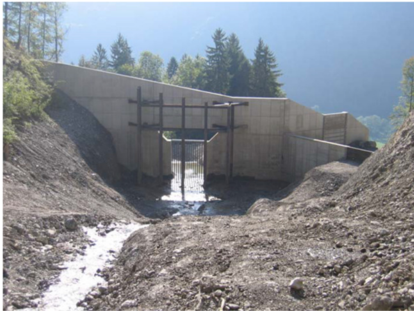
Retention basin after modification
