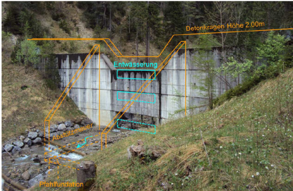
Modification measures planned in the flood protection project Source: Theiler Ingenieure AG
