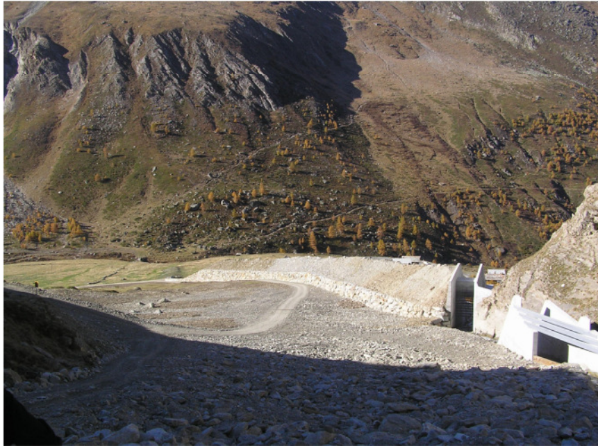
Outlet dam (right), screen dam (left of outlet dam) and deflection dike with deposition area (left)
