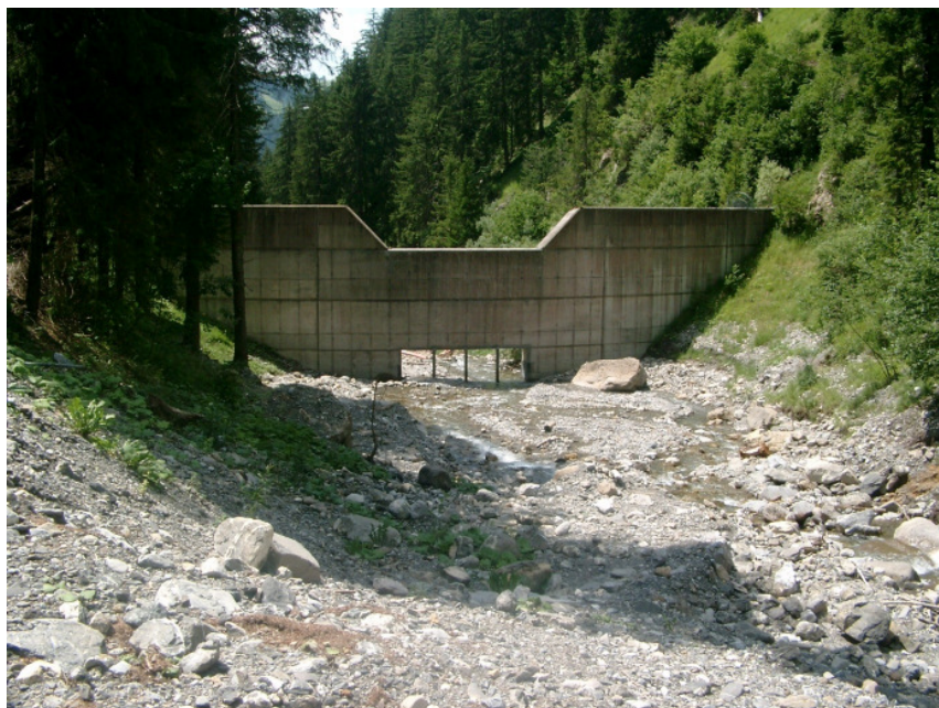
Existing arch dam, retention basin of Betelriedgraben
