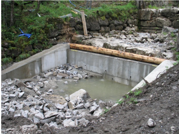
Construction of a subsidiary dam
