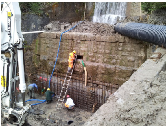
Pre-concreting Source: canton of NW
