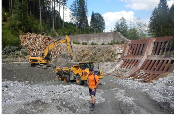
Fig. 9: Operation can also cause high efforts, for example retention basins have to be emptied from time to time
