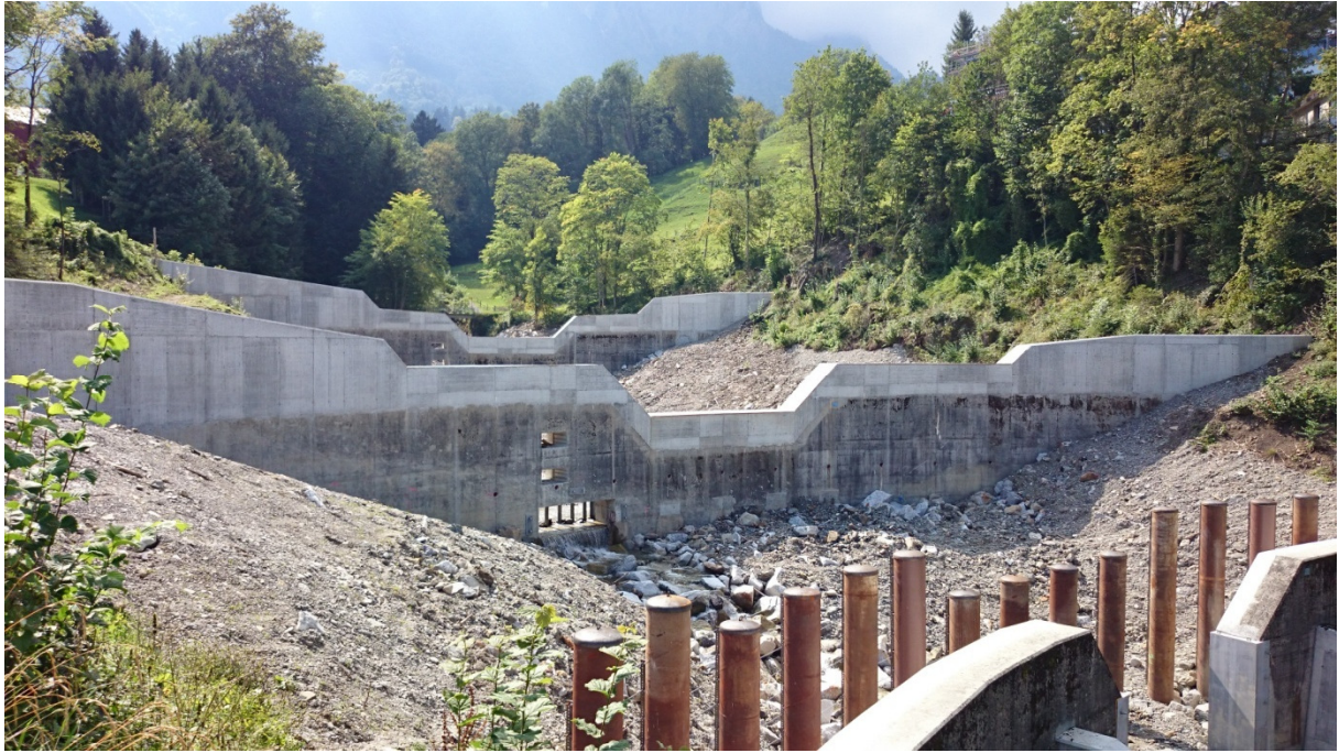
View over the finished construction
