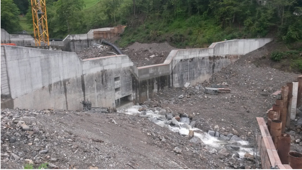
Arch dams 1 and 2 after modification
