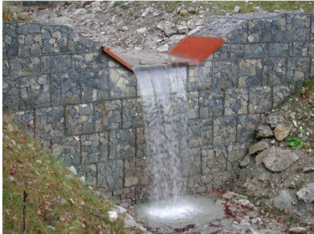
Gabions would quickly get destroyed due to abrasion especially in the spillway section. Therefore, “easy to replace” steel plates cover the endangered part of the dam construction. Example Talgraben, Lkr. Bad Tölz-Wolfratshausen, Bavaria
