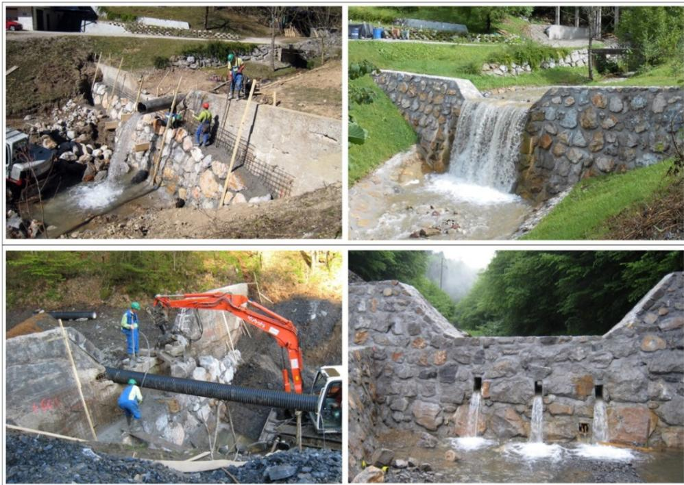
One of the solutions to maintain the design functionality of decrepit old dams is the reinforcement of building massive supporting stone constructions in front of old structure, anchored and connected with the existing one and actually working like one object (two examples from the torrents Mačkov graben and Prošča, photo: Hidrotehnik, Slovenia)
