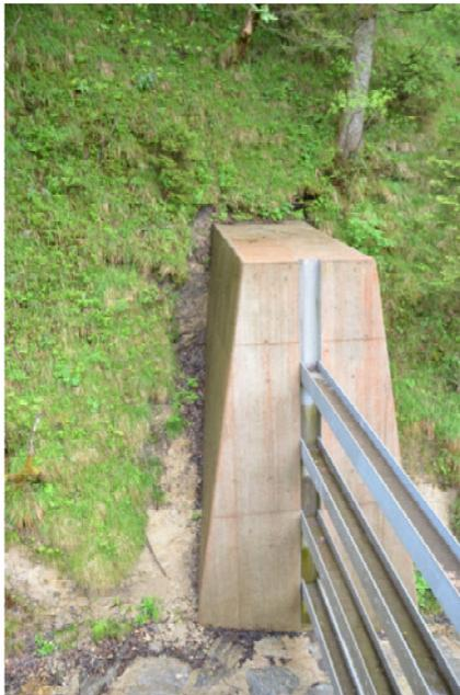
The vertical distance of the steel beams in this retention dam can easily be changed. So this construction can be adapted to further experience without having to rebuild it. Example Maigraben, Lkr. Rosenheim, Bavaria
