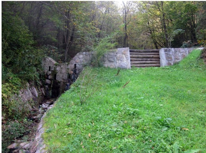
New boundary conditions demand upgrading of functionality of existing protection structures – a common measure is raising protection dams. On the photo there is such an example from the torrent Lučno, with additional adapting of structure with manageable passage (closed with removable wooden trunks) for local owners who have to occasionally gather the woods from the forested headwaters (photo: Hidrotehnik, Slovenia)
