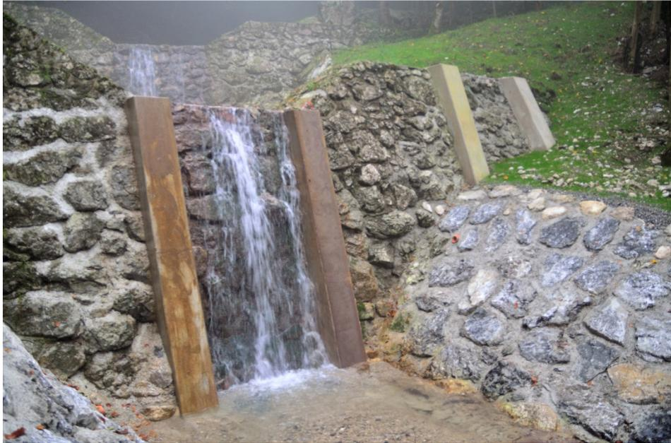
The old rock dam was not stable enough. Instead of its total replacement, it was reinforced by back-anchored concrete columns. Example Maigraben, Landkreis Rosenheim, Bavaria
