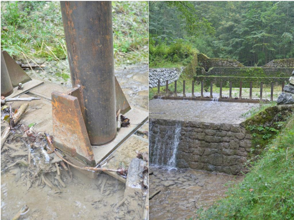
The steel columns of this woody debris entrapment rake can easily be fixed in different distances to each other. So this construction can be adapted to further experience without having to rebuild it. Example Maigraben, Lkr. Rosenheim, Bavaria
