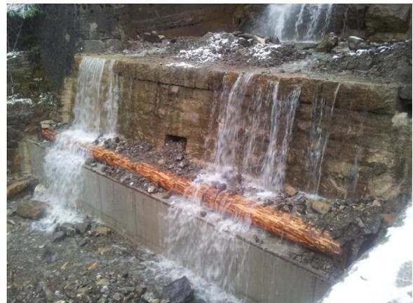
Finished pre-concreting and coverage with log
