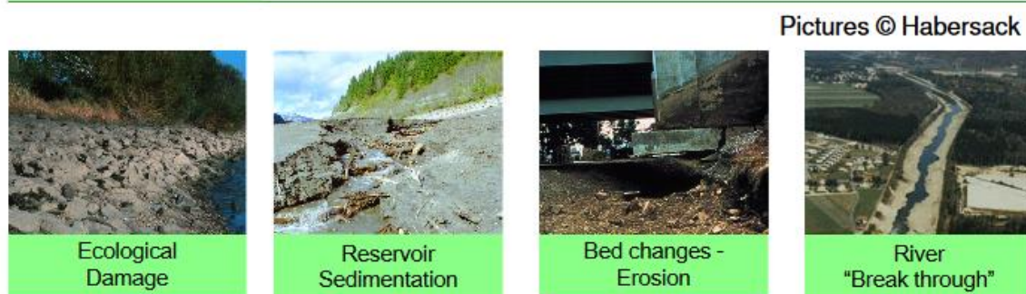
Figure 12 - Sediment surplus or deficit effects (Source: Schwaiger K., 2012 4 )
