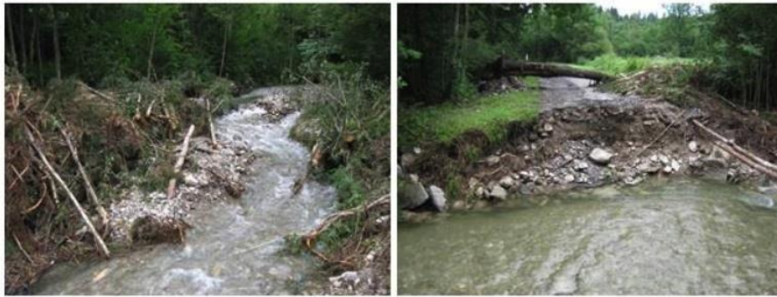
Figure 26 - Wood log jam destroyed a bridge; also several check dams were damaged
