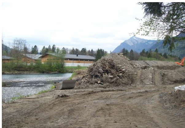
Figure 16: Example of works carried out on the opposite riverbank to remobilise aggraded material
