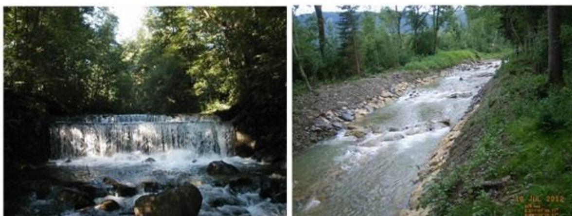
Figure 12: Before and after; a 3 m high check dam is replaced by a 120 m long ramp
