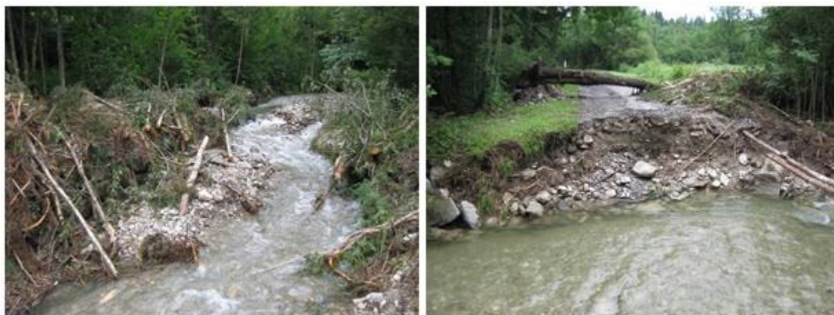
Figure 11: Wood log jam destroyed a bridge; also several check dams are damaged
