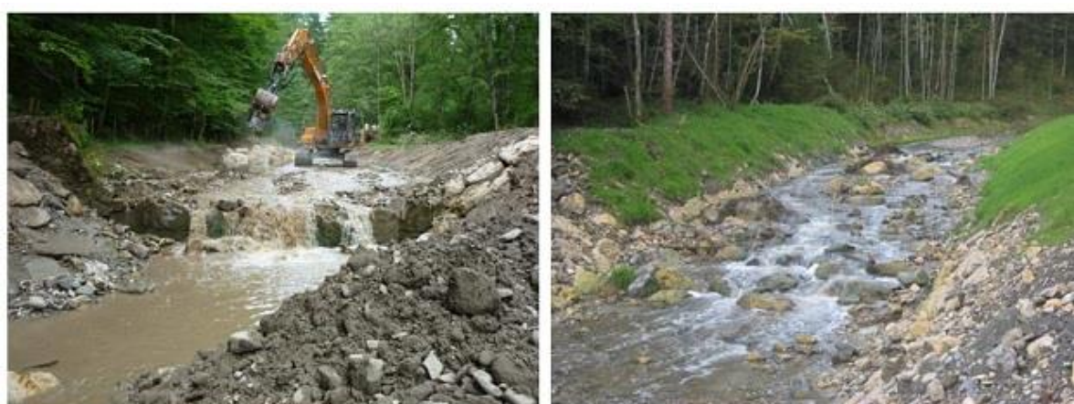
Figure 13: During and after the reconstruction (ramp with a height of 1.6 m and a length of 70 m)
