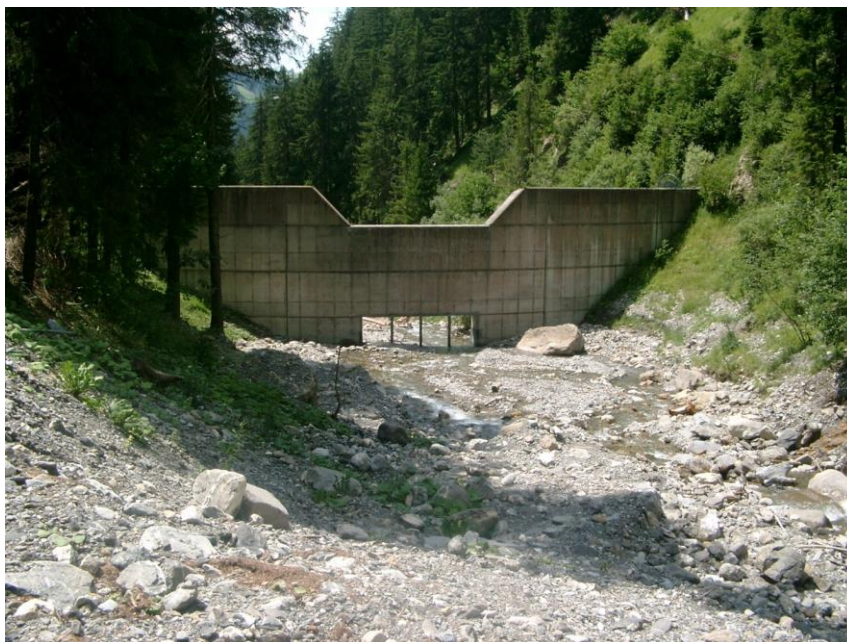
Existing arch dam, retention basin of Betelriedgraben
