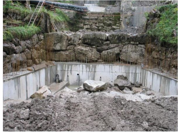
Pre-concreting and training structures
