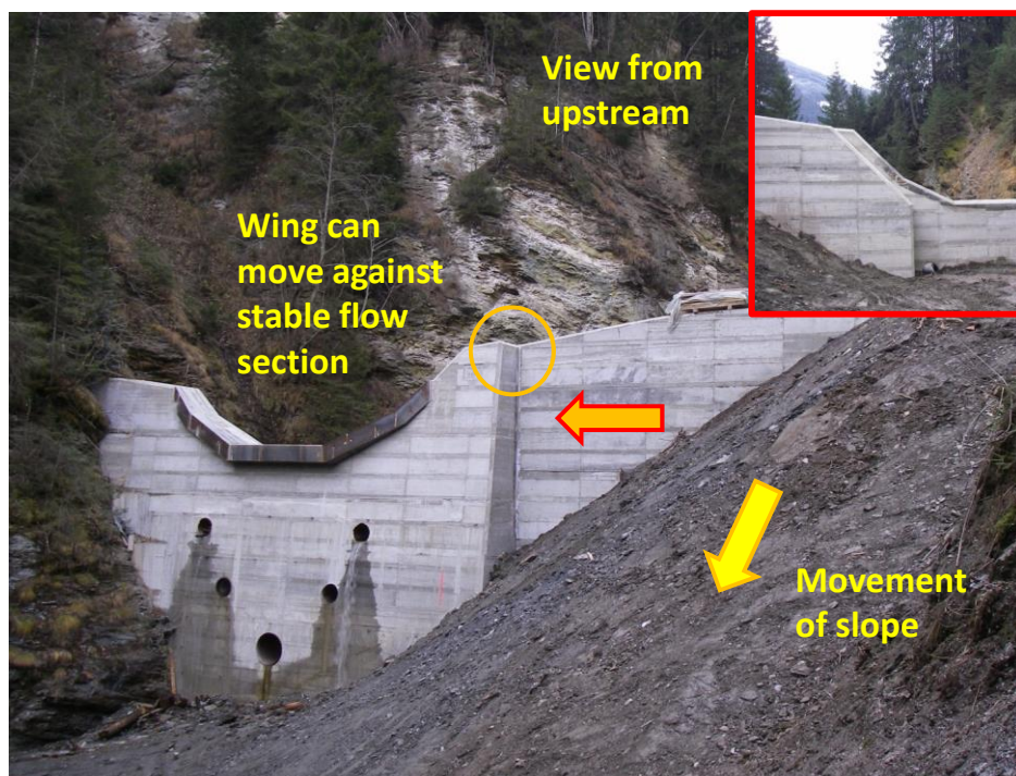
Check dam with a slidable wing to balance lateral mountain pressure, Source: die.wildbach (Salzburg)
