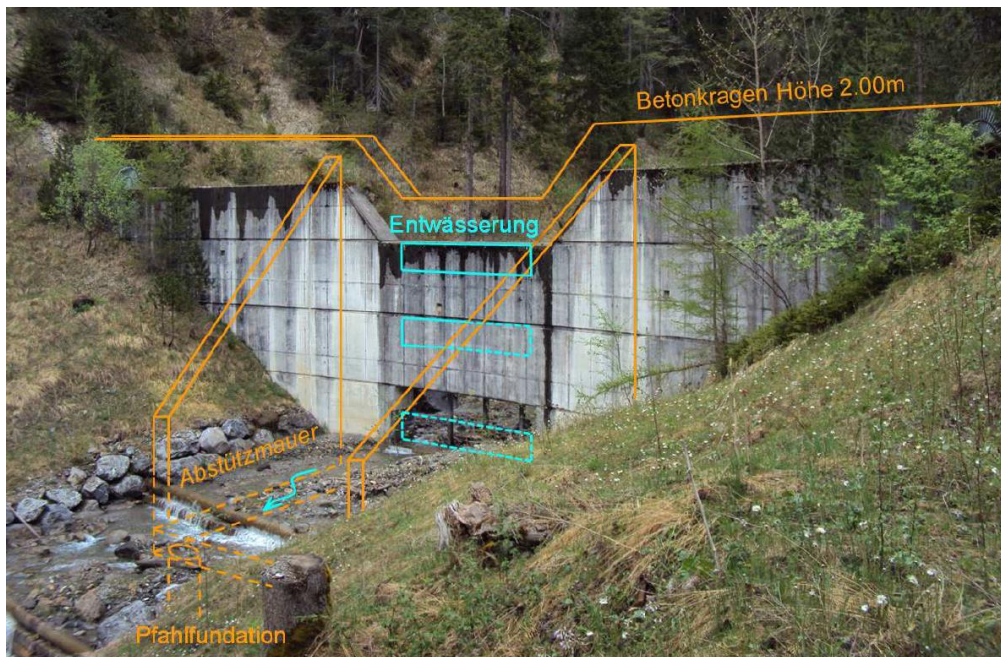
Modification measures planned in the flood protection project Source: Theiler Ingenieure AG
