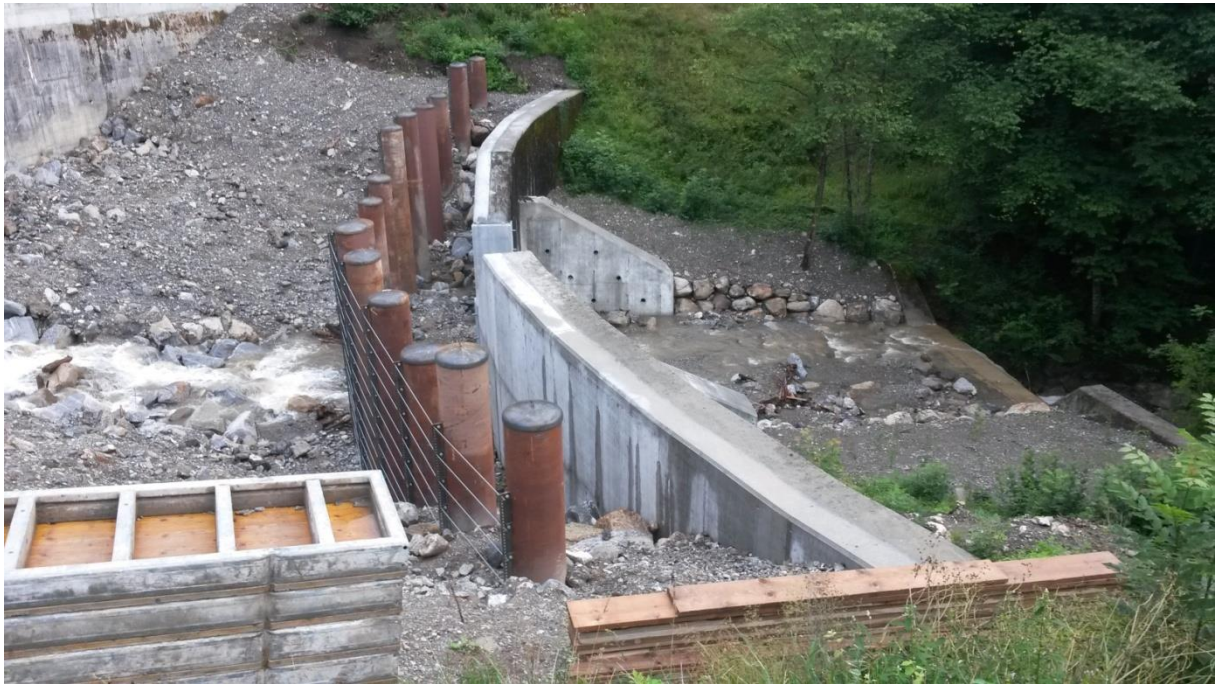
Modification of arch dam 3 for retention of woody debris
