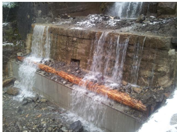
Finished pre-concreting and coverage with log Source: Kanton NW
