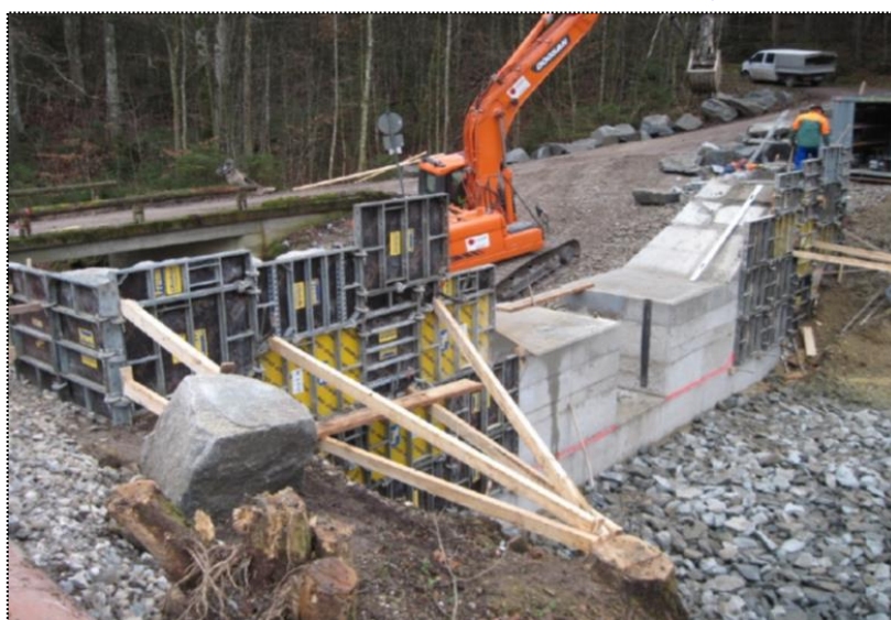
Fig. 17: Building of the new sediment control dam (Picture: WWA Weilheim)
