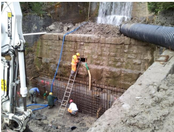
Pre-concreting Source: Kanton NW
