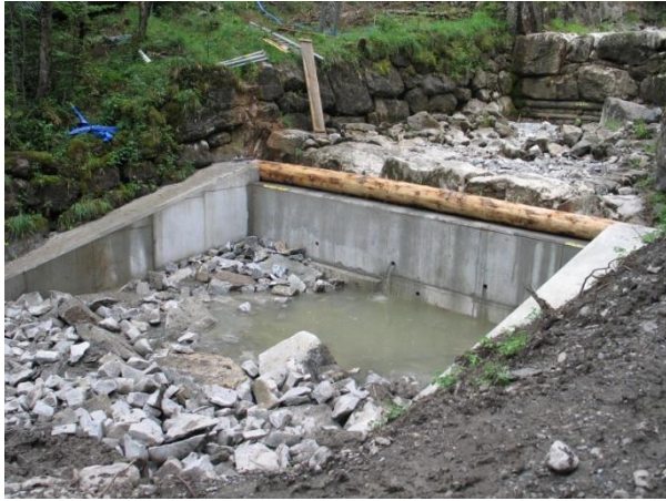
Construction of a subsidiary dam
