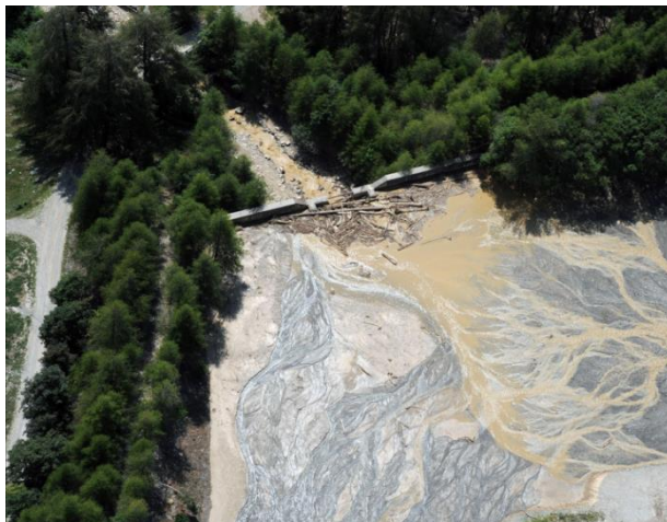
Fig. 21: Gadria creek: Details of the clogging mechanisms (i.e. through driftwood and solid material) of the check dam openings and the consequent full aggradation of the disposition basin.
