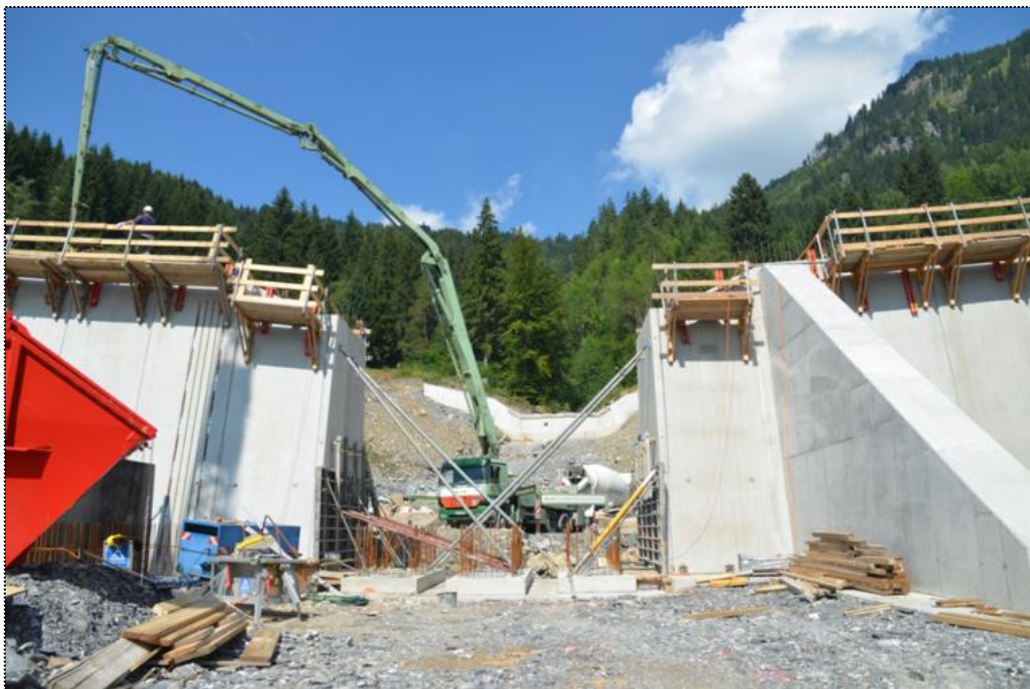
Fig. 10: Realization of a debris flow control structure in the torrent Zillenbach, municipality Hindelang, Oberallgäu (Picture: WWA Kempten)
