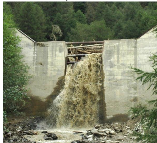
Fig. 21: Gadria creek: Details of the clogging mechanisms (i.e. through driftwood and solid material) of the check dam openings and the consequent full aggradation of the disposition basin.
