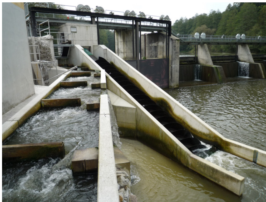
Fig. 2 Reversed water auger © State Office for Water Management Deggendorf
