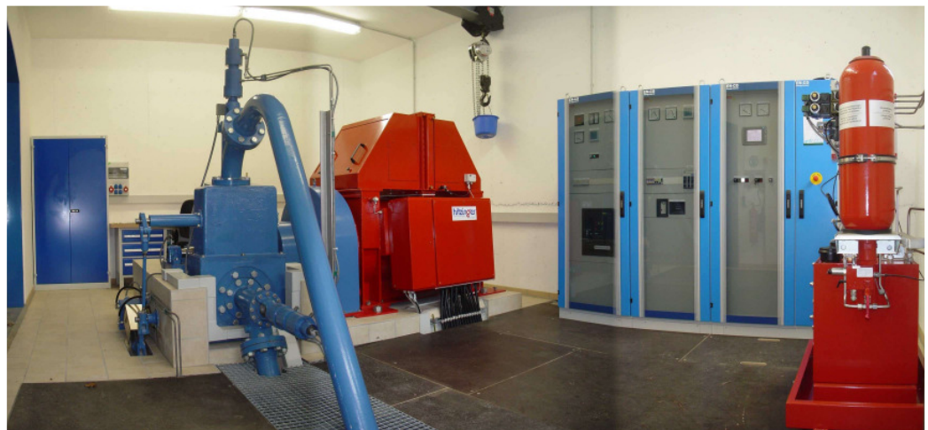
Fig. 4: Interior panorama (Hydroelectric generating set with Pelton turbine, synchronous alternator and electrical equipment) © Gemeindewerke Garmisch-Partenkirchen
