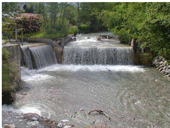
Figure 7: Weirs and dams can fragment habitats and be obstacles for fish migration by causing an interruption of the longitudinal river continuity (© H. Mühlmann, BMLFUW)
