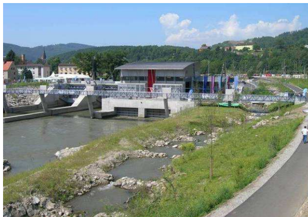
Figure 8: Near-natural fish pass at a smaller river in Austria. Fish migration aids reduce the negative effects of the fragmentation of rivers (© Verbund)
