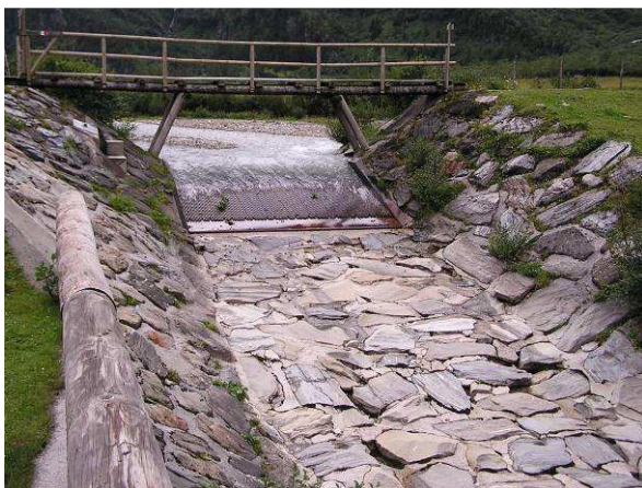
Figure 9: No water – no life. Insufficient residual water beneath a Tyrolean weir for water abstraction for hydropower generation is causing an obstacle for fish migration and a loss of habitats (© H. Mühlmann, BMLFUW)
