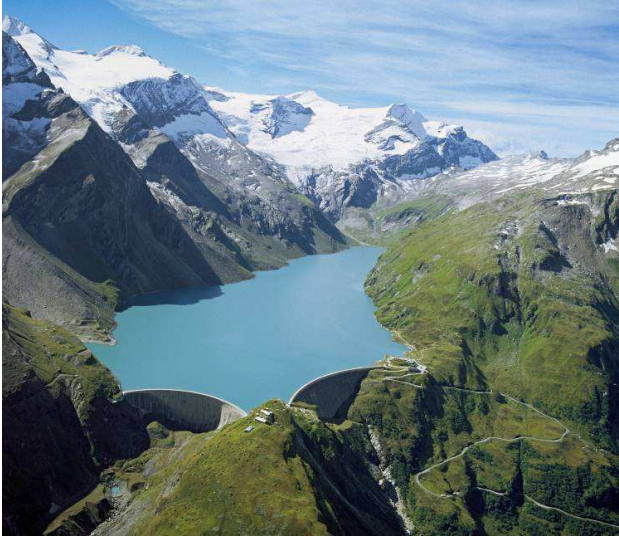
Figure 12: Alpine reservoirs and impounded river stretches – reduced flow velocities lead to increased depositions of fine sediments while periodical flushings can cause severe negative impacts of downstream river stretches (© Verbund)
