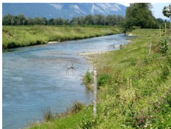
Figure 29: Part of the restored stretch of the Inland Canal. The structural elevation and the adjustment of the flow velocity and water depth promote the development of feeding and breeding areas for water birds, small animals and various fish species. © M. Fasel
