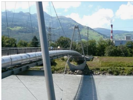
Figure 28 The new Energy Bridge across the Rhine, between the canton of St. Gallen and Liechtenstein, serves as a bicycle path and carries the steam pipe from the KVA (background, right). © M. Fasel
