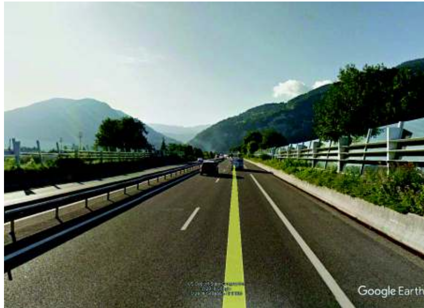
Illustration 14: view from the A40 showing acoustic insulation around Scionzier-Cluses
