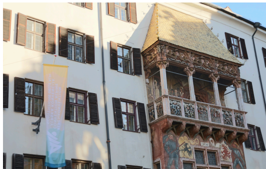
Goldenes Dachl, housing the Innsbruck office © Permanent Secretariat
