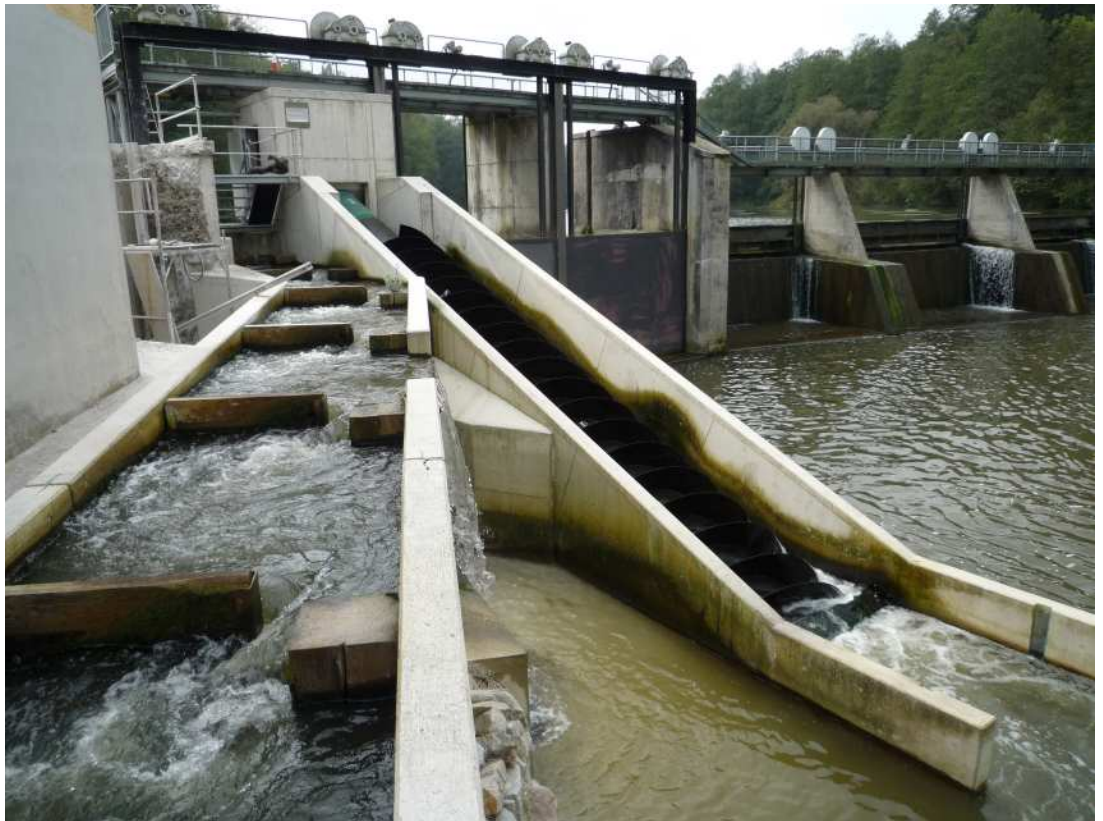
Figure 25: Reversed water auger
