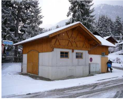
Figure 20 and Figure 21: Power house © Bavarian Environment Agency
