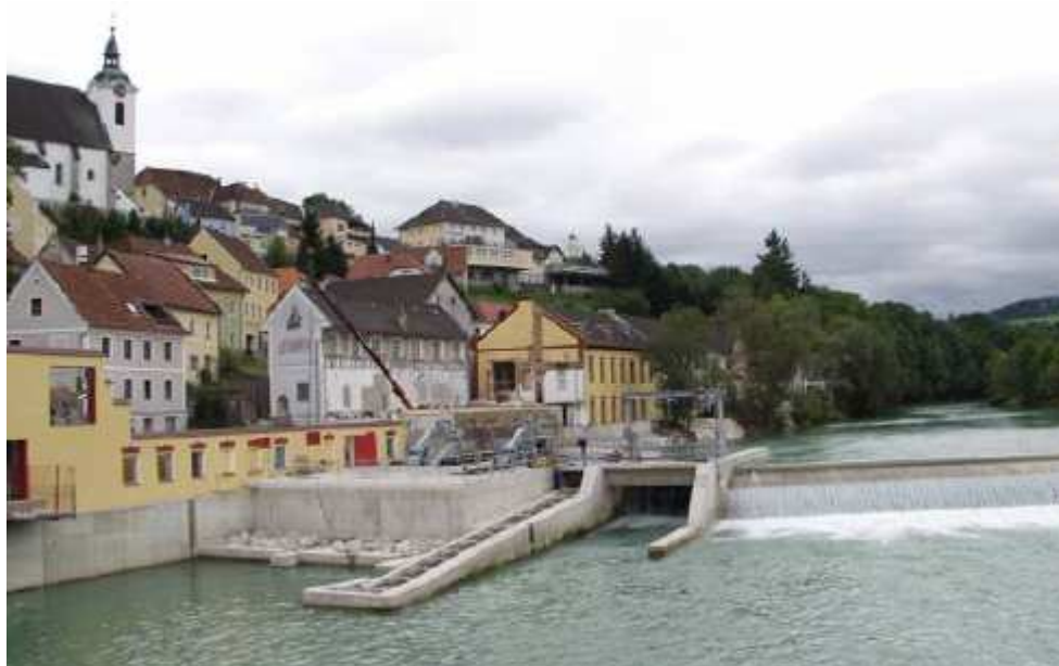
Figure 7: Vertical slot SHPP Steinbach
