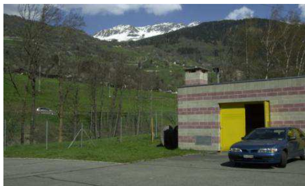
Figure 47: Water intake in Verbier
