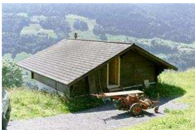
Figure 43: The small hydropower plant of Troistorrents. © MHyLab
