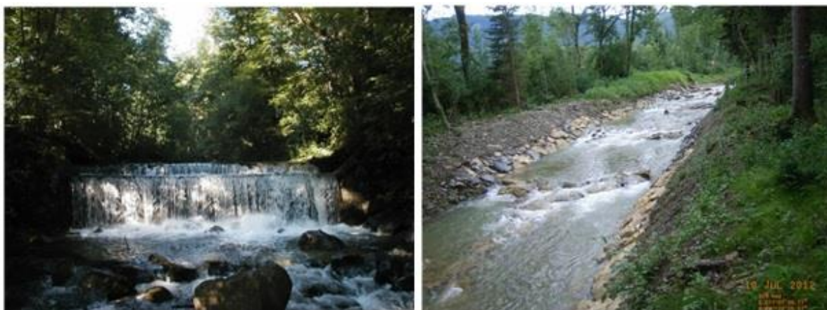
Figure 12: Before and after; a 3 m high check dam is replaced by a 120 m long ramp
