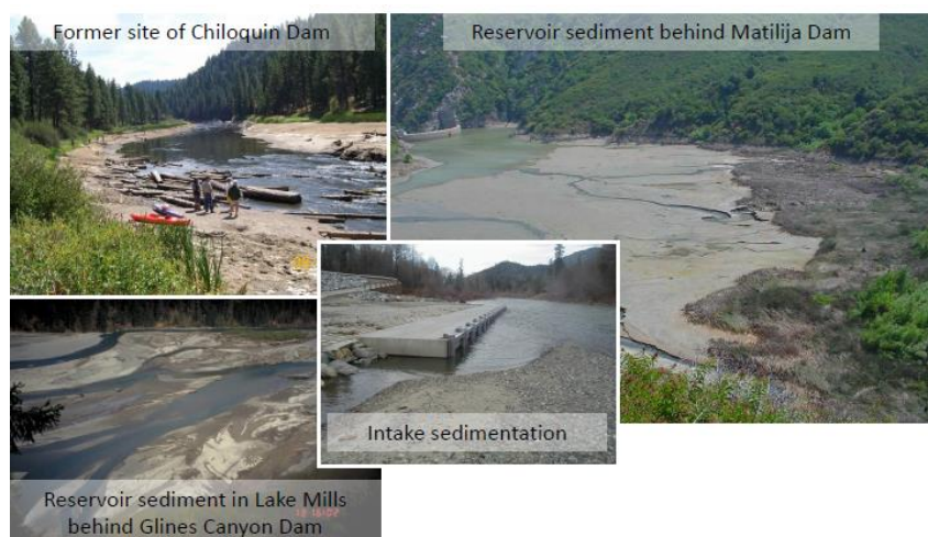
Figure 18 - Possible impacts of the sediment in a river
