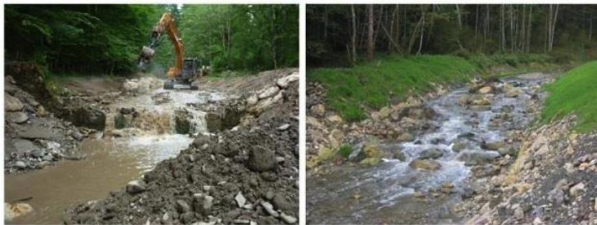
Figure 27 - During and after the reconstruction (ramp with a height of 1,6 m and a length of 70 m)
