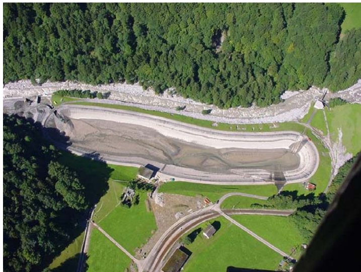
Figure 8: Surveys of defence measures must always consider what happens in the case of overload. Flood control reservoirs and outflow corridors must be created in case structural measures prove insufficient for the scale of the incident (photo: Swiss Air Force, Switzerland).
