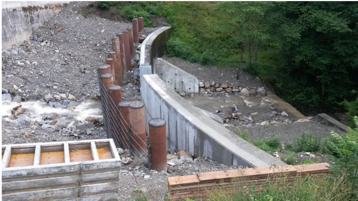
Modification of arch dam 3 for retention of woody debris
