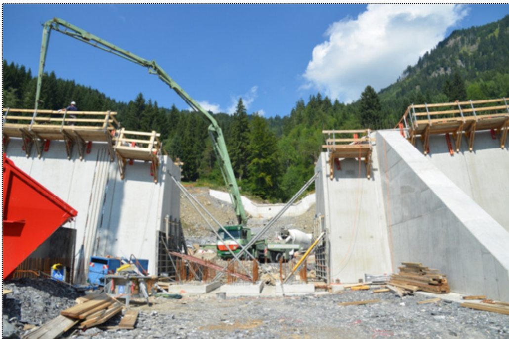
Fig. 10: Realisation of a debris flow control structure in the torrent Zillenbach, municipality Hindelang, Oberallgäu (Picture: WWA Kempten)
