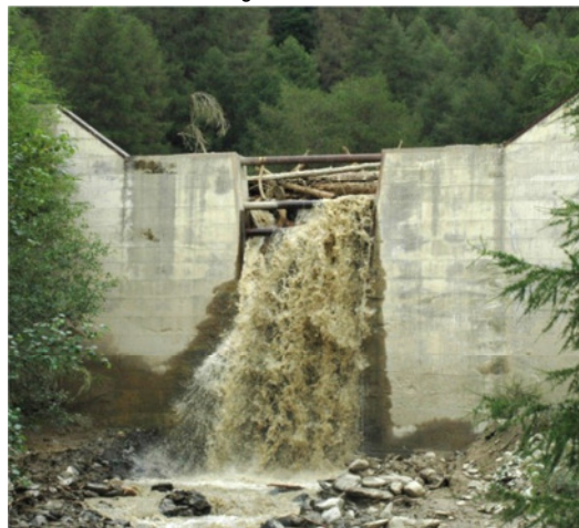
Fig. 21: Gadoria creek: Details of the clogging mechanisms (i.e. through driftwood and solid material) of the check dam openings and the consequent full aggradation of the disposition basin.
