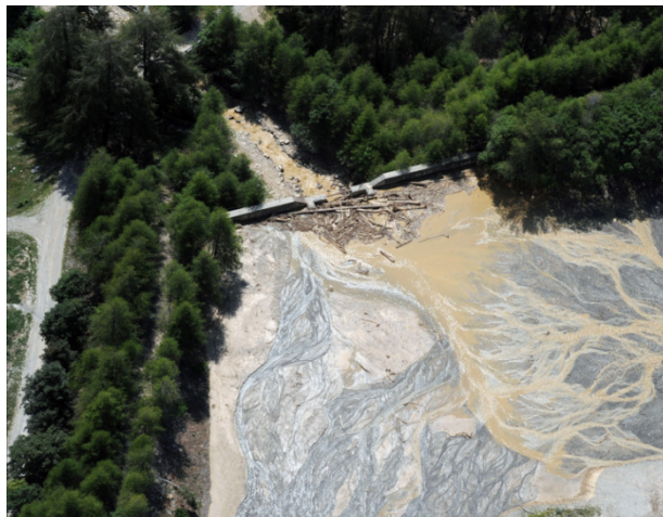
Fig. 21: Gadoria creek: Details of the clogging mechanisms (i.e. through driftwood and solid material) of the check dam openings and the consequent full aggradation of the disposition basin.
