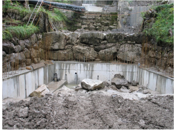
Pre-concreting and training structures
