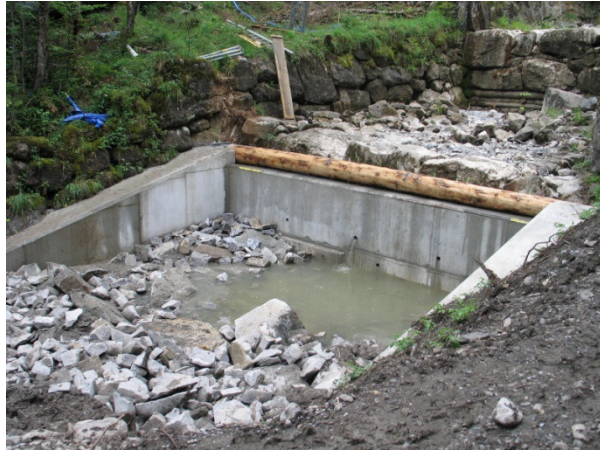
Construction of a subsidiary dam
