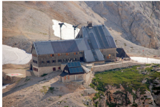
Solar panels & collectors and wind turbine at Kredarica hut
